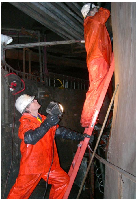
Sidewall acousto ultrasonic-echo technique inspection
