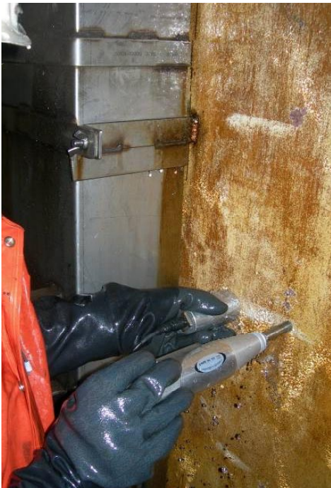
Blast furnace acousto ultrasonic-echo inspection
