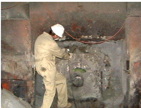
Tapping block inspection
