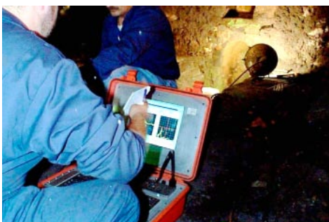
Acousto ultrasonic-echo taphole inspection
