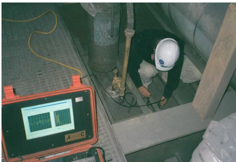
Reheat furnace anchor brick inspection
