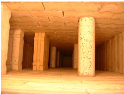
Bake furnace flue wall interior
