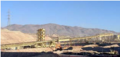
The materials handling systems (8,800 tph) designed and construction managed by Hatch for the Escondida Norte & E3 project in Chile included a new primary crusher station, overland and distribution conveyors and surge and distribution silos
